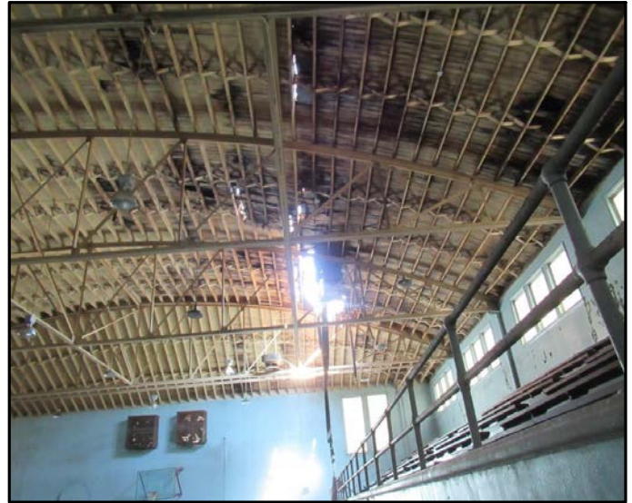
Light seen through the roof
