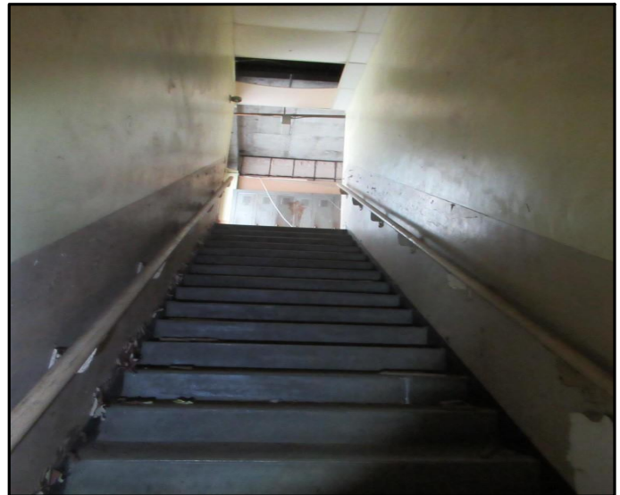
Stairway to second floor
