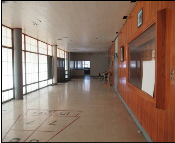
Front main lobby
