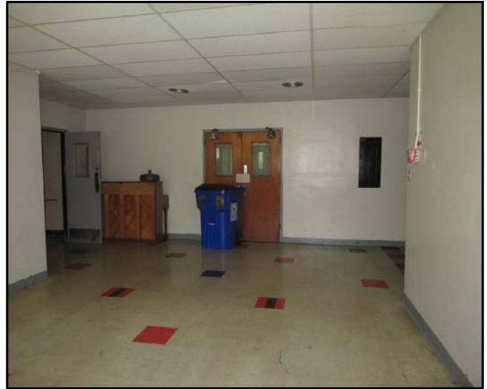
Entrance north side of Bldg
