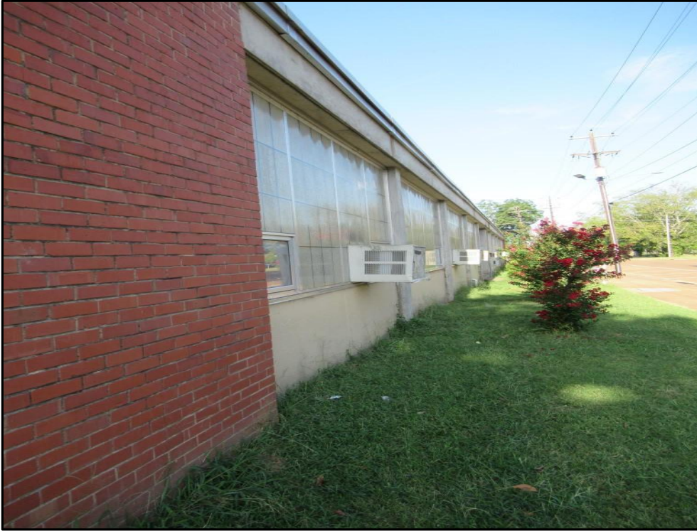
Looking along left side of bldg
