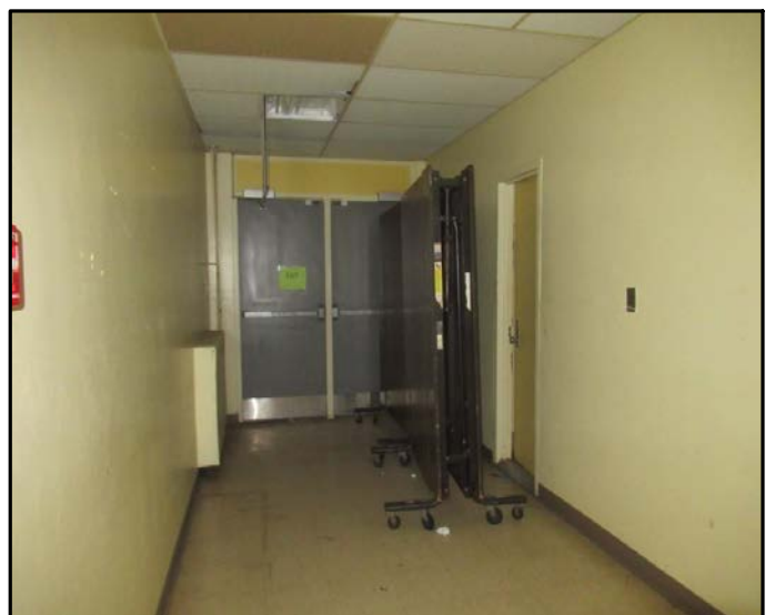
Exit door in hallway
