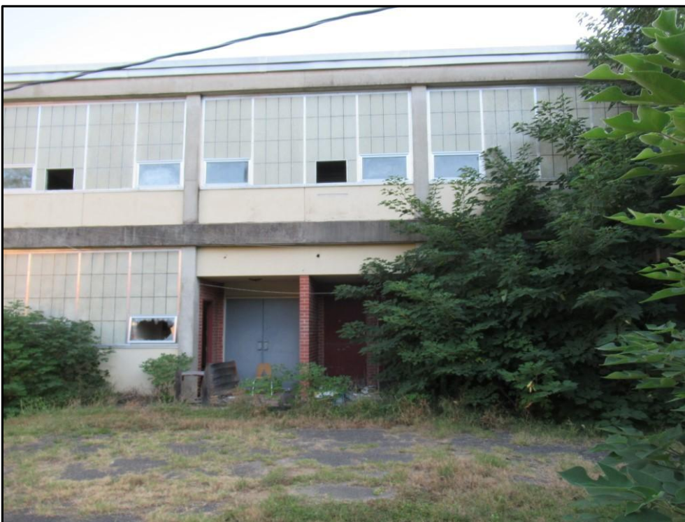
Partial view of rear of bldg
