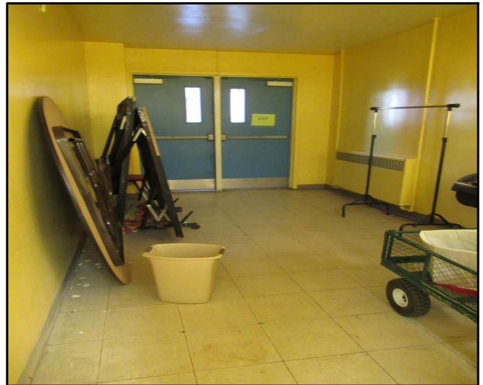
Hallway to rear entrance
